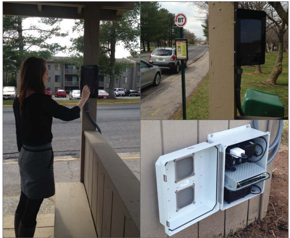
FIGURE 3-17 KIOSK INSTALLED AT BLACKSBURG TRANSIT BUS STOP
