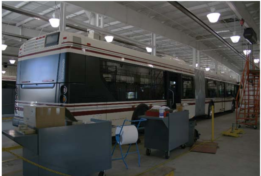
FIGURE 2-6 BLACKSBURG TRANSIT 60 FT. (18.2 M) BUS IN SERVICE BAY
